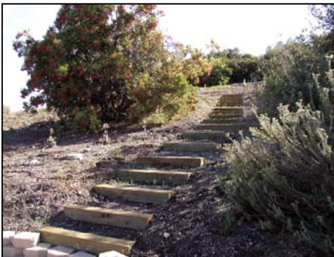
Newly installed steps and habitat at George F Canyon.
